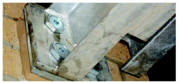
**BoxBolt** is a fully tested and approved blind connection solution for connecting to hollow section steel or where access is restricted to one side only. The **BoxBolt** is suitable for use with rectangular, square and even circular hollow sections. The features a hexagon head design to aid installation with a standard wrench. It allows it to be installed with our unique **BoxSok™** installation tool for when installation time needs to be kept to an absolute minimum.
